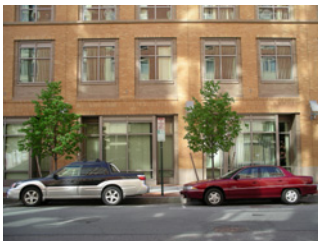
Individual window openings break up the facade and add interest at the street level.
