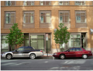
Buildings windows should be individual openings in the façade, not continuous bands of windows.
