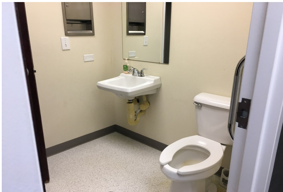
Rest Rooms (5 Total)
