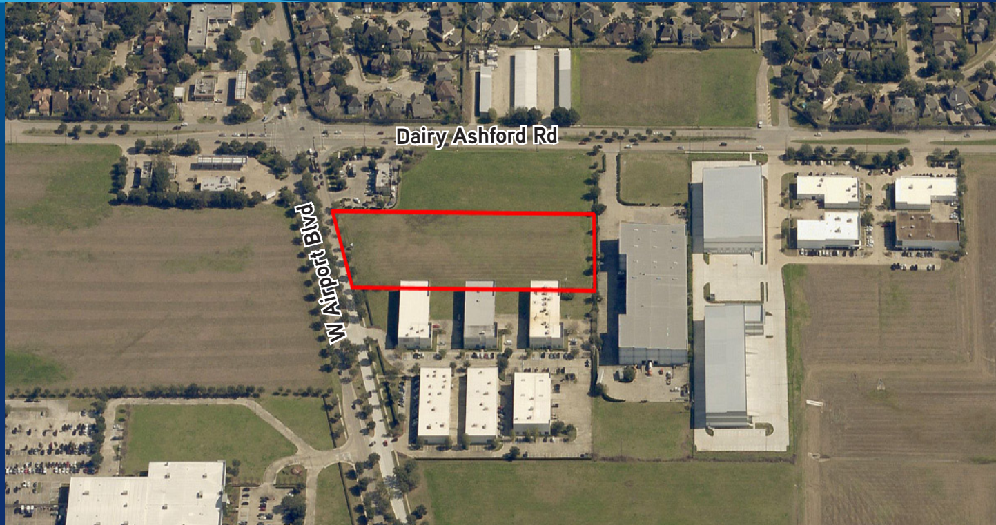
VIEW OF SITE LOOKING EAST
