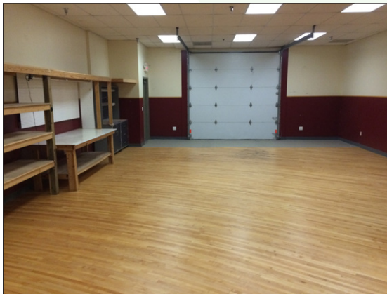
Endcap with overhead door
