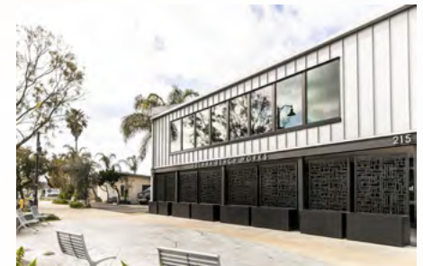
EXTERIOR PATIO FOR SUITE 100
