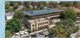
1020 Alma 1020 Alma Street 25k sf Under Construction Tenants to Include: Hillspire LLC, Schmidt Family Foundation, Schmidt Ocean Institute
