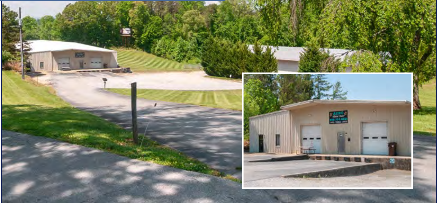
Twin Springs Business Park; Inset: close-up of 145, showing drive-in door and dual-height loading dock
