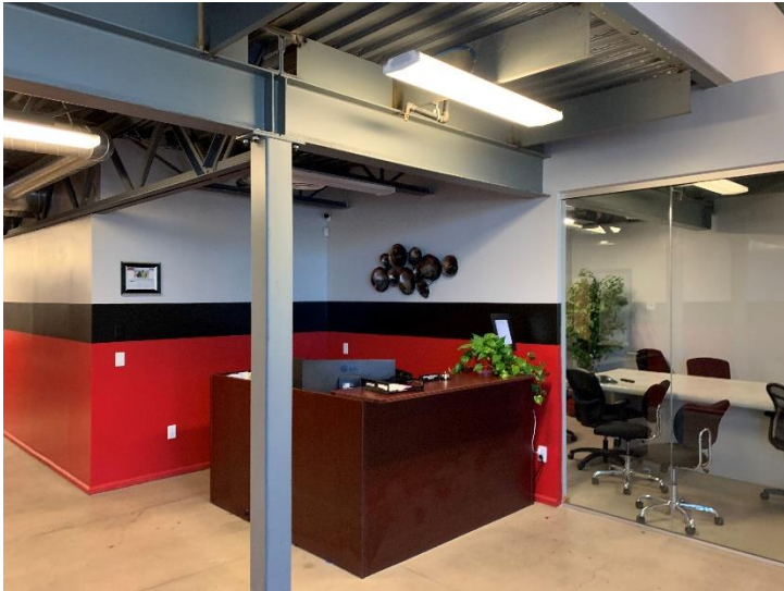
High-image office build-out
