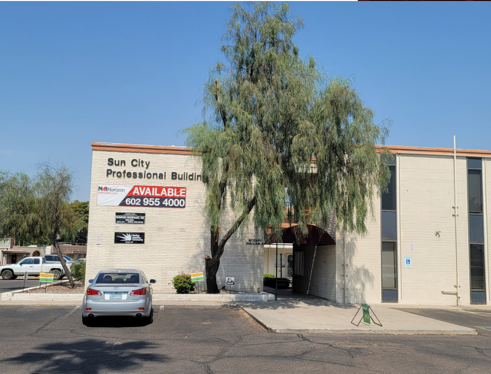
East facade & parking
