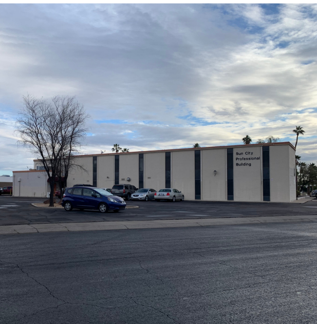
West facade & parking
