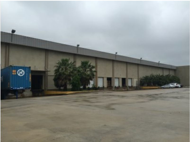
FRONT LOADING AREA
