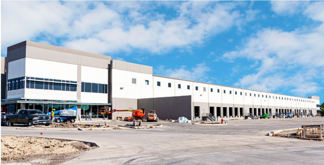
* Building 1 ( \pm 260,000 SF): Finalizing windows and landscaping. Delivery expected 08/2019.
