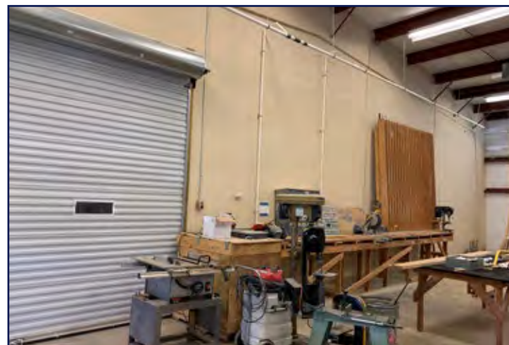
10 Brandy Branch Rd - warehouse partition wall
