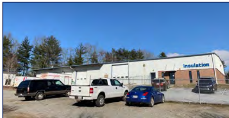
8 Brandy Branch Rd - exterior
