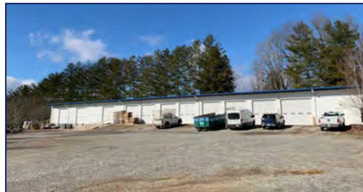
10 Brandy Branch Rd - exterior
