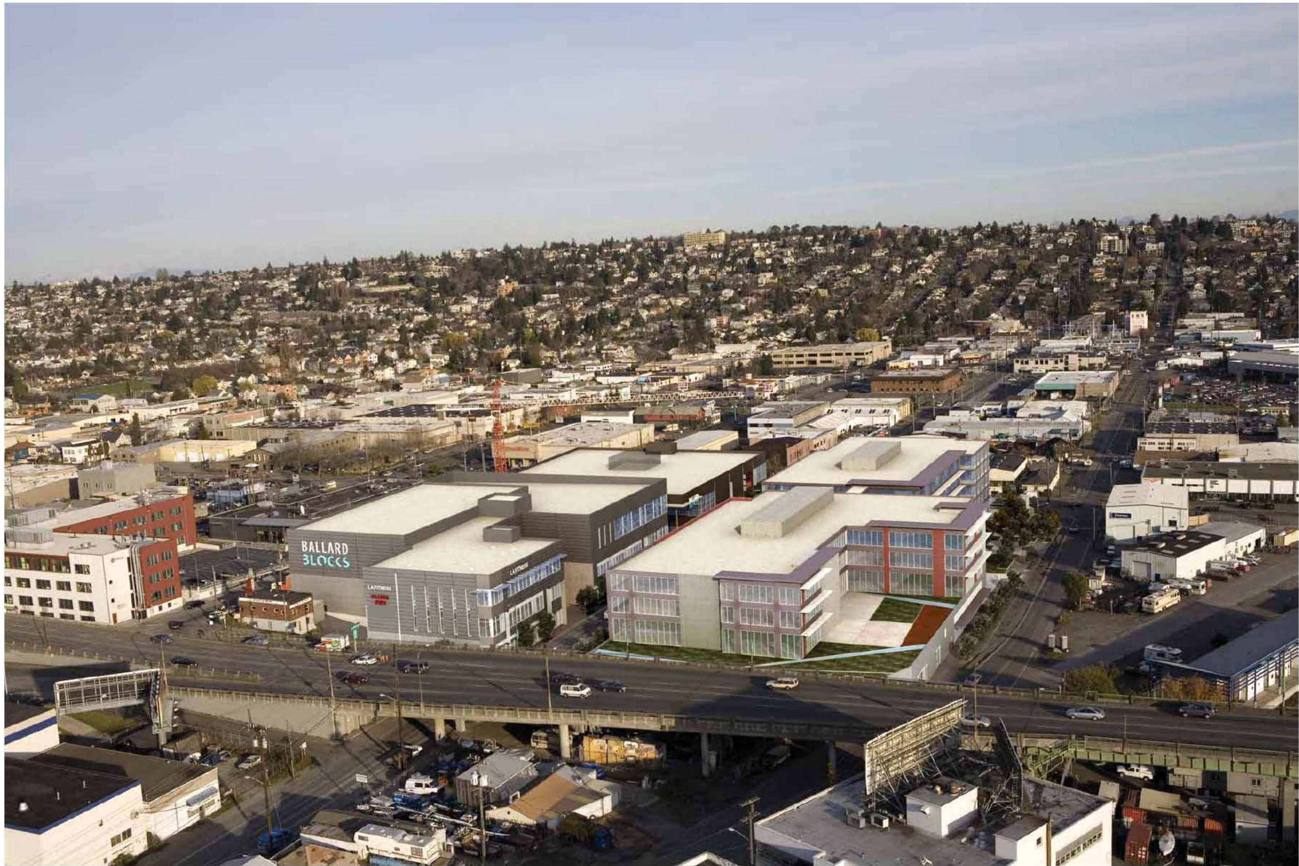
BALLARD BLOCKS north east view
