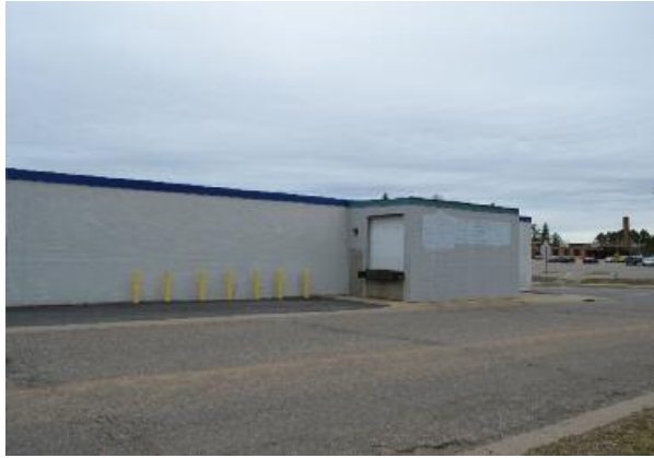
West Loading Dock / OH Door
