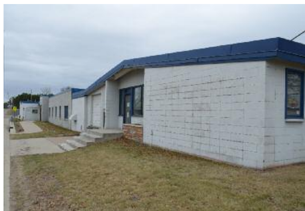
Entire Building (View from NE Corner)
