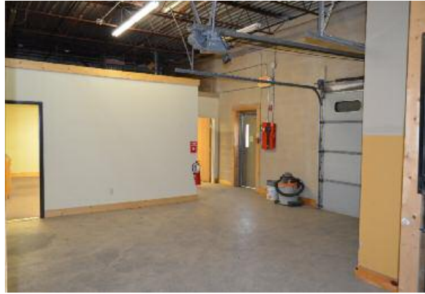
East OH Door & Entrance
