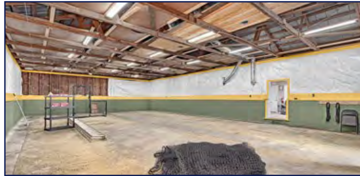
Small building - warehouse interior
