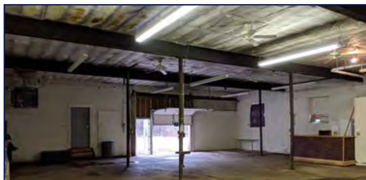
Large building - basement, looking toward drive-in door
