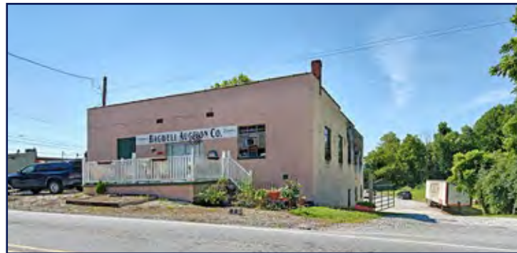
6,720 SF building backs up to Fanning Bridge Rd
