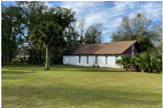
Building Exterior and Grass Parking
