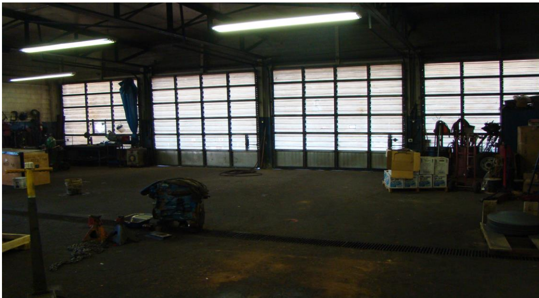
WAREHOUSE LOOKING TOWARD ROLL-UP DOORS TO NORTH
