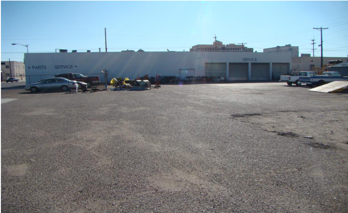
MOSTLY PAVED PARKING LOT/YARD SPACE NORTH OF BUILDING
