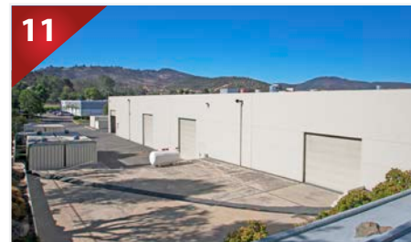
Grade Level Doors/Dock Platform
