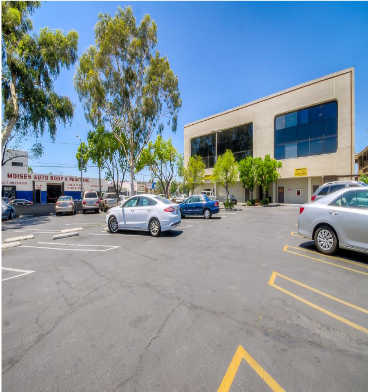
Free parking in the back. Reserved parking spaces for tenants.
