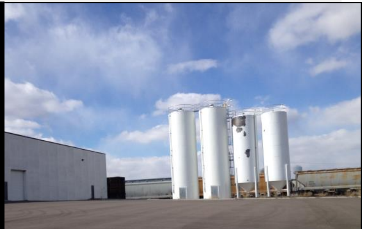
4.75 acres: 4 silos, rail & outdoor storage
