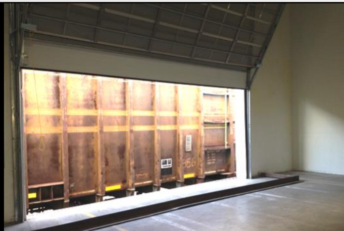
Rail Access Door (20'Wx10'H) w/screen
