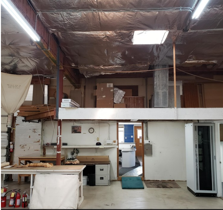
Warehouse and Mezzanine
