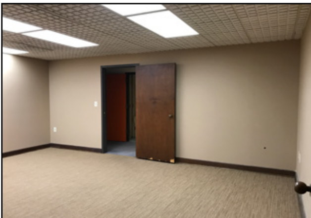
2nd Floor Office
