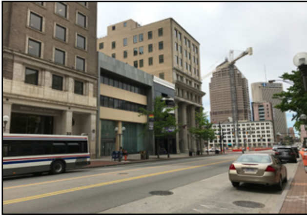
Exterior facing North
