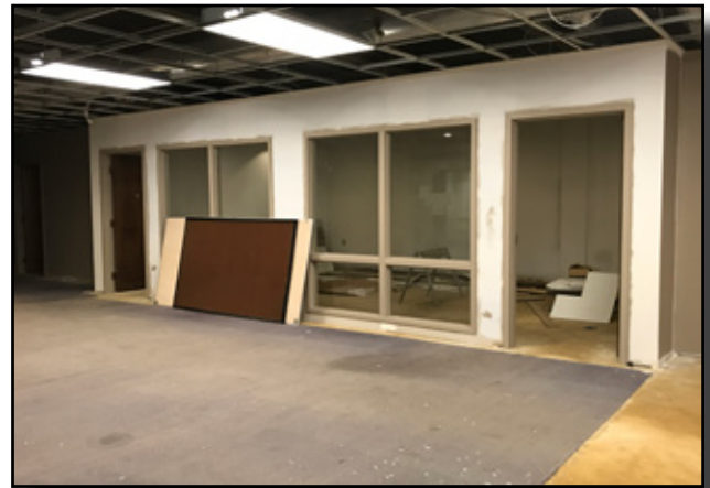
3rd Floor Office
