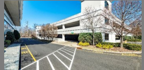
COVERED PARKING DECK
