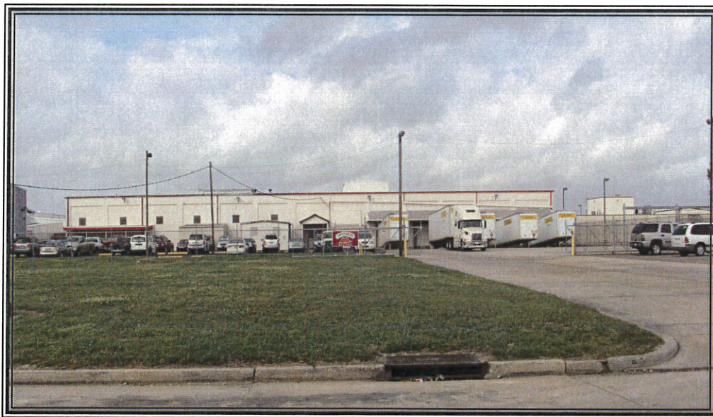
Access to back of building
