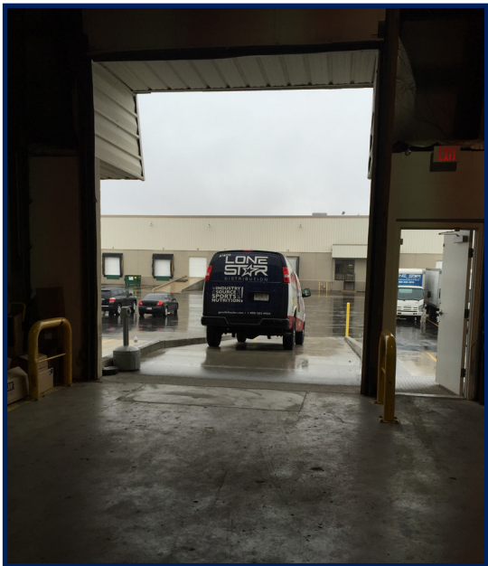
Interior View of Doors
