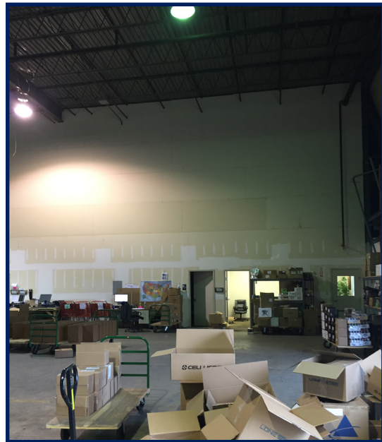
Interior View of Main Floor
