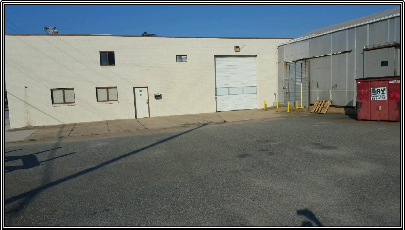
Side of building with grade level door 14' x 12'
