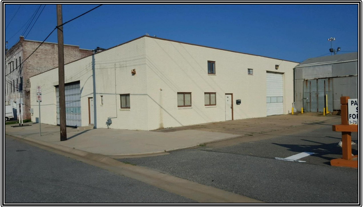
Front and side of building
