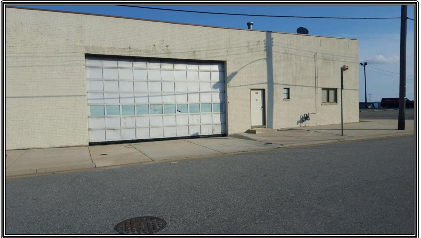
Front of building Overhead door is 24" high and 14' x 24'
