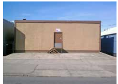
EAST SIDE OF BUILDING
