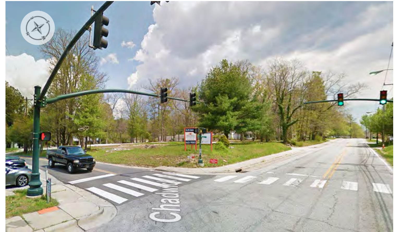
At intersection of US25/Greenville Highway and Chadwick Avenue - lot has been cleared of major structures
