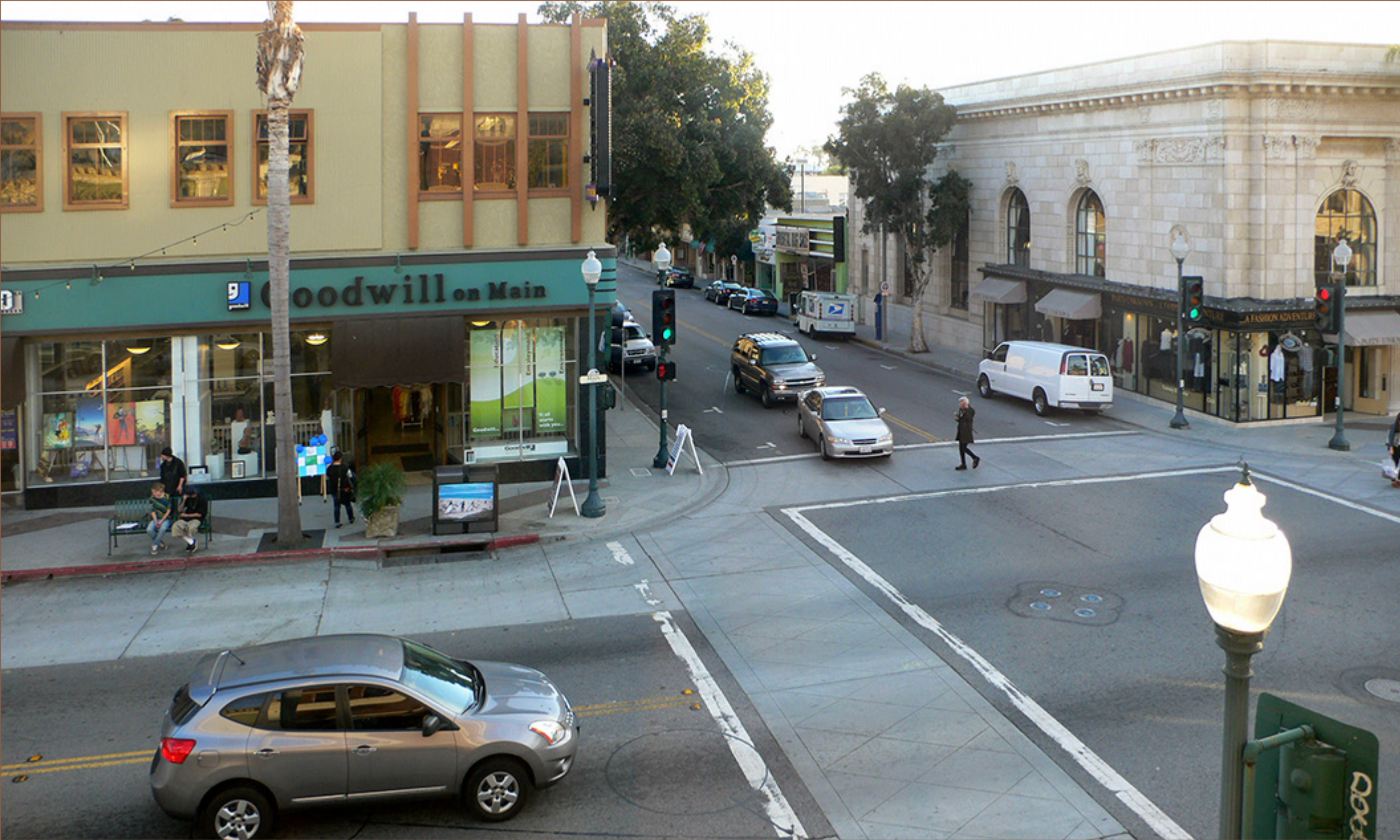
upstairs building corner view
