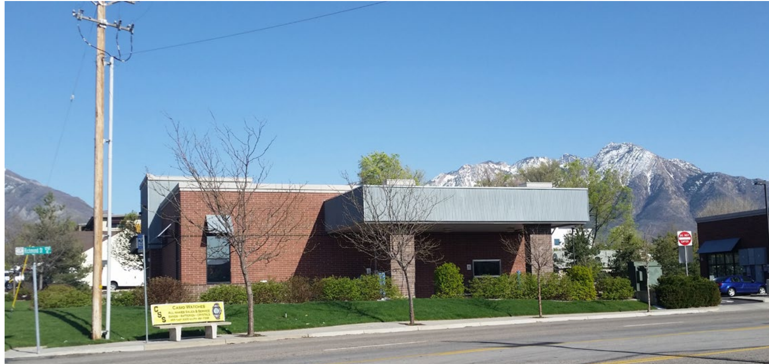
West Side of Building: Excellent visibility from Richmond Street and Harmons.
