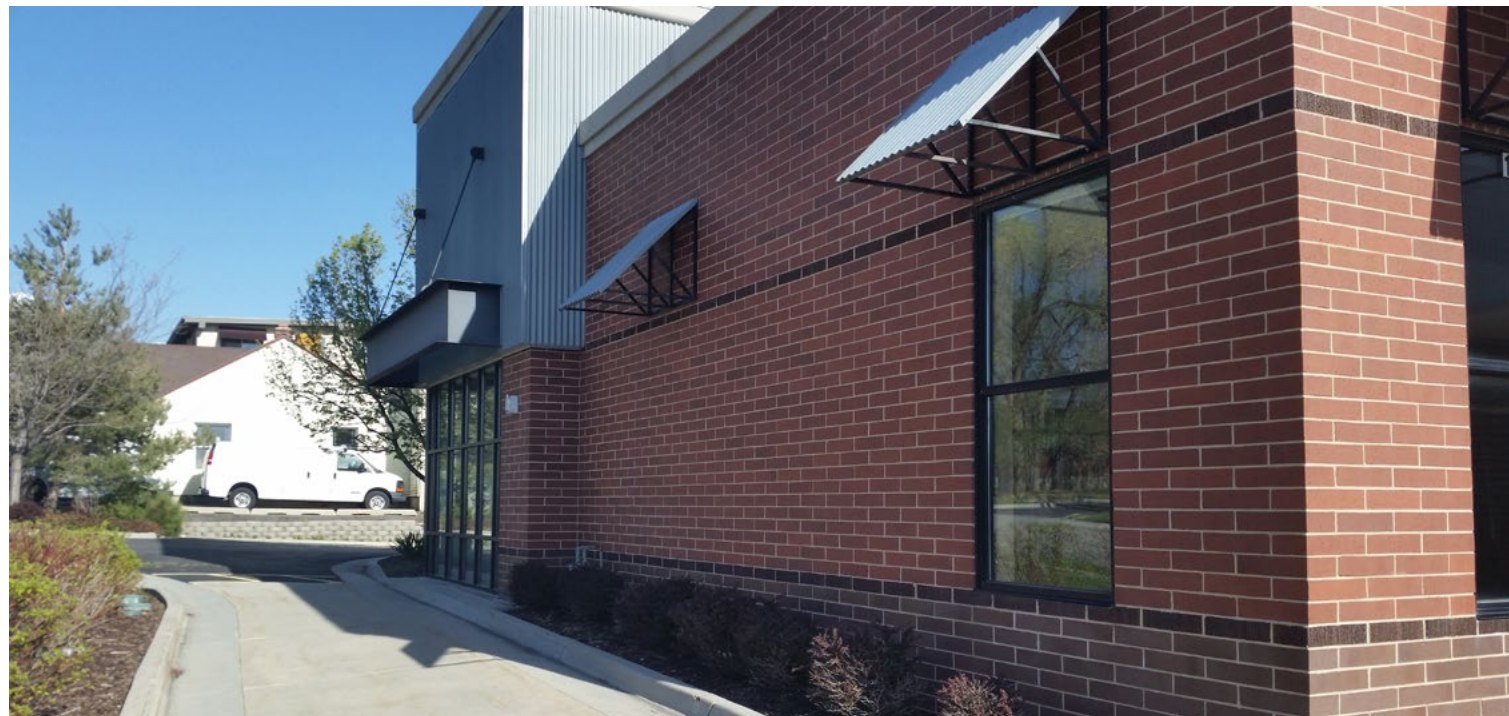
East Side of Building: Could be converted to a patio area.
