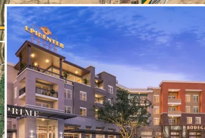
AGRITOPIA EPICENTER Breaking ground Fall 2017
