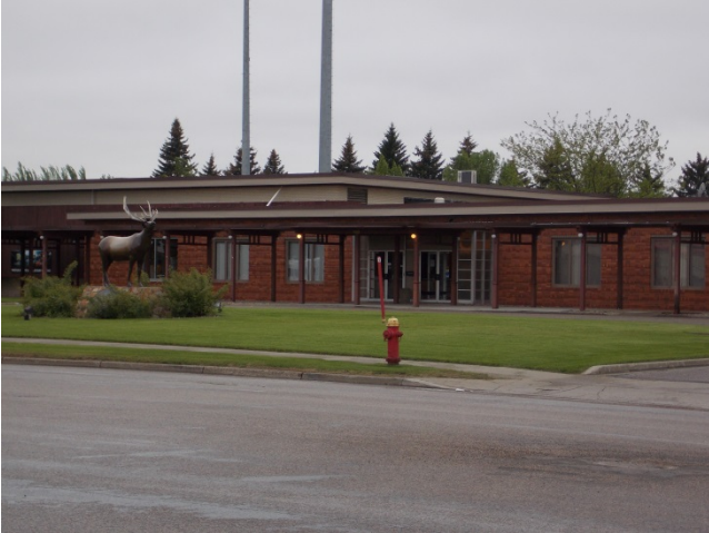
Elks Lodge Directly Adjacent to the South
