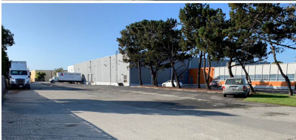
Large Rear Parking Area with Additional Loading Docks
