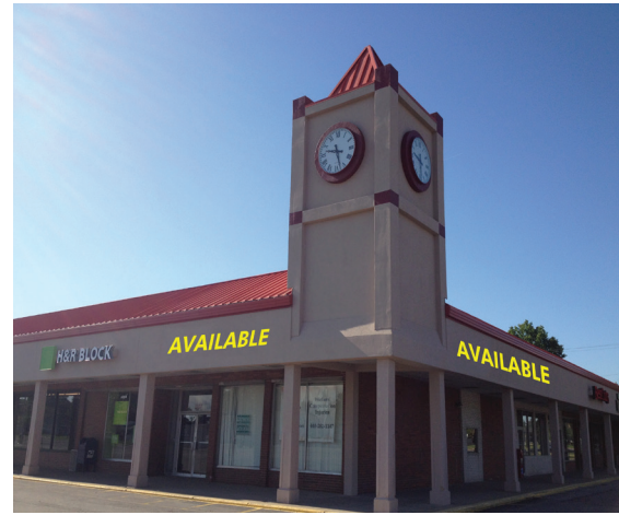
1,170 SF corner unit along Oberlin Ave
