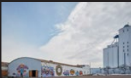
1325 Quincy, Minneapolis (Quincy Hasll Building)
