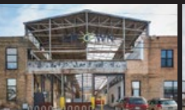
Crown Center, Minneapolis
