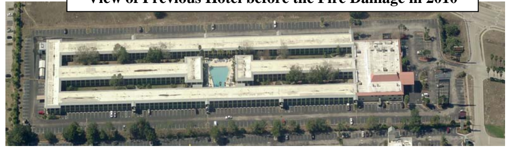
View of Previous Hotel before the Fire Damage in 2010
