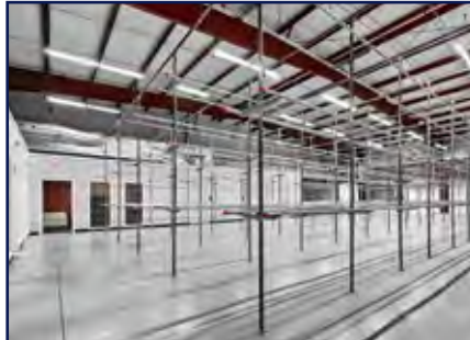
Warehouse from front
