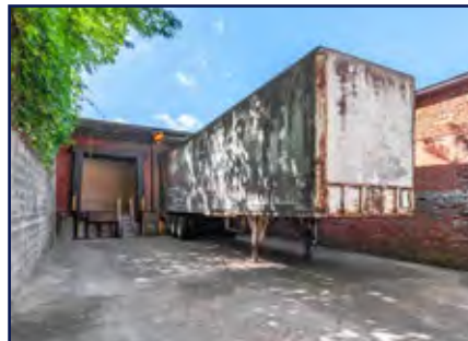
Exterior loading dock; trailer included
