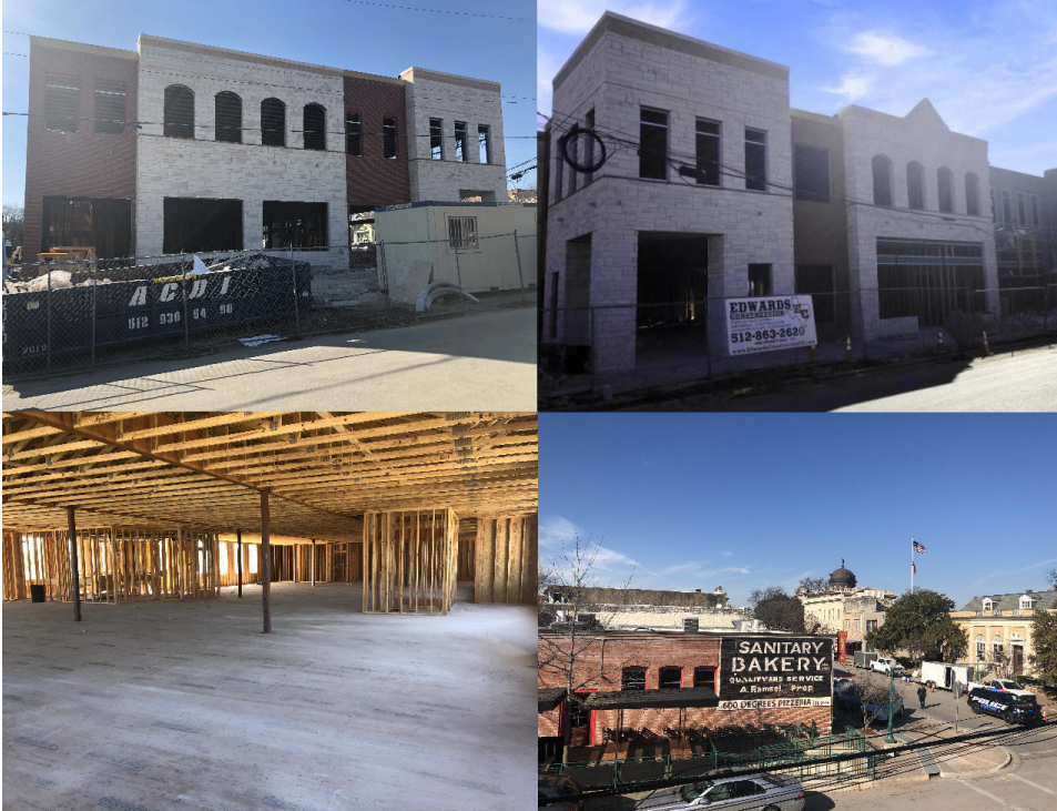
INTERIOR AS OF JANUARY 8, 2020
