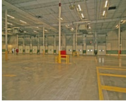
10 FULLY EQUIPPED 9' X 10' DOCK DOORS
