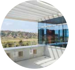
THIRD FLOOR BALCONIES AND FIRST FLOOR PATIOS
