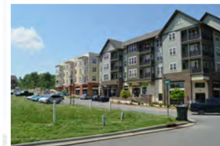
RIVER DISTRICT APARTMENTS
