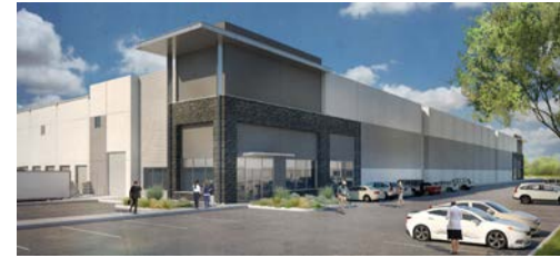
Jackson Shaw Class A Industrial Under Construction 320,000 SF
