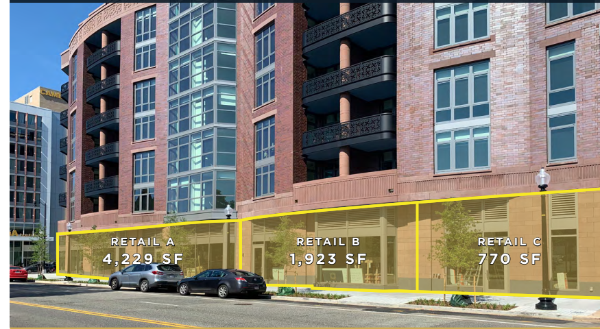
VIEW NORTH FROM 9TH STREET
