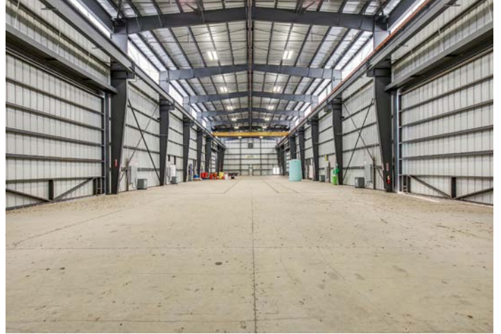
Building 2: 10-Ton Crane
