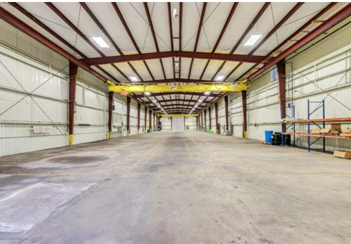
Building 4: (1) 10-Ton + (1) 5-Ton Crane
