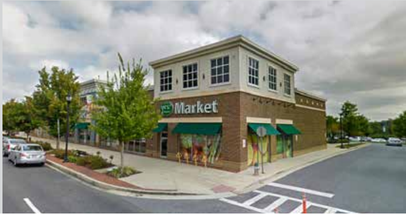
BALTIMORE AVENUE, LOOKING NORTHEAST
