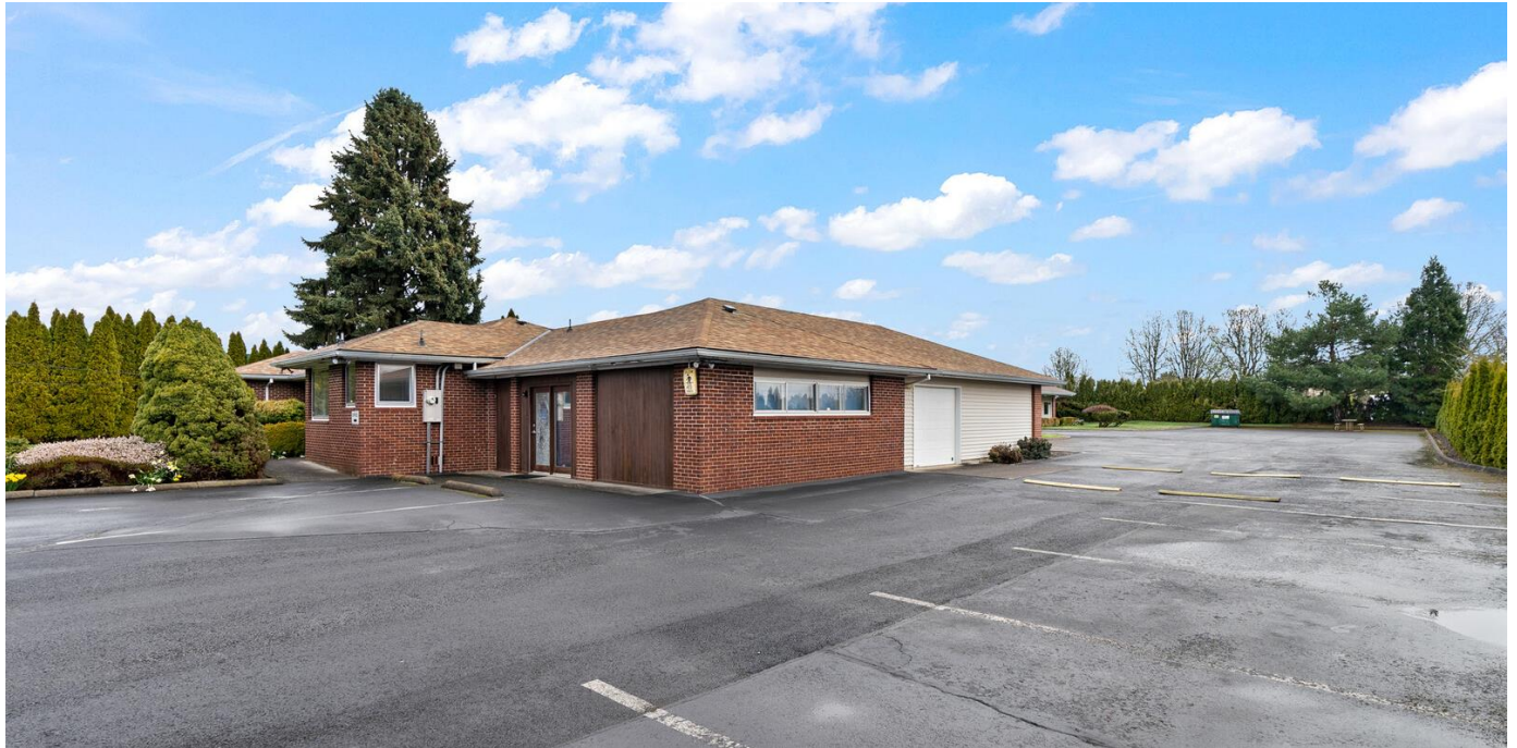
Front building (office and associated storage) 3,263 SF
