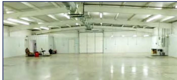
Climate-controlled section, including restroom and shop area
