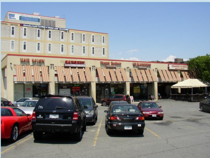
Exterior showing retail amenities
