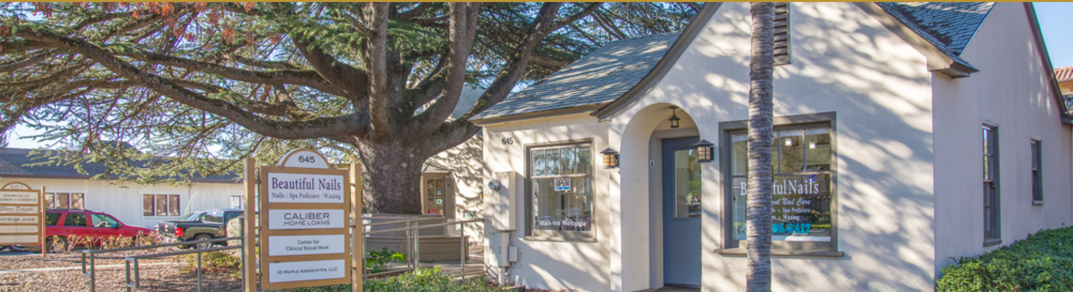
Front of 645 Broadway building
