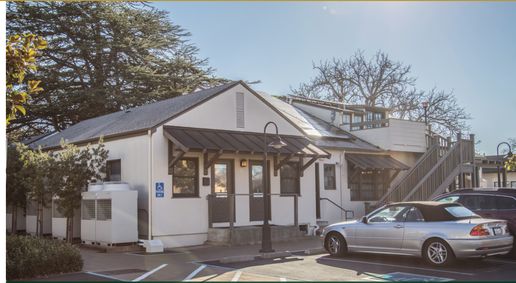
Rear of 645 - 651 Broadway building.
