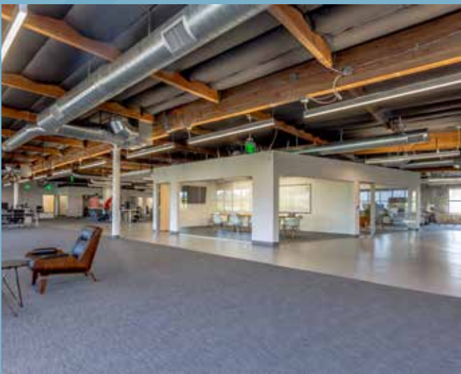
OPEN TO STRUCTURE CEILINGS
